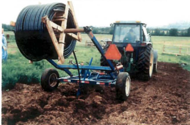
Pasture pipeline plow laying pipe at Rainey Ranch.
