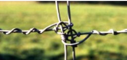
Wrap-splice: Give yourself 4-6" of wire past the end stay. Lay the end wires together and wrap the ends together with pliers
