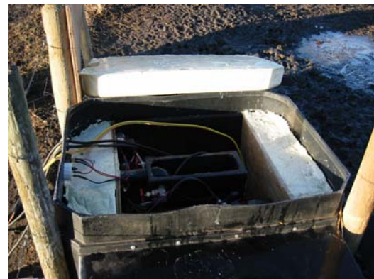
Insulation is about 2' thick around batteries and bowl to prevent the water in the bowl from freezing.
