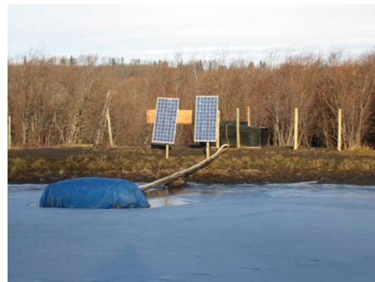
Hogberg's winter CAP system. Two 105 watt panels. Tarped barley bale to keep pump from freezing.
