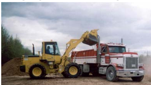
Loading the custom spreader truck
