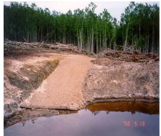
Horst David built a ramp with geo-grid plastic and crushed gravel.
