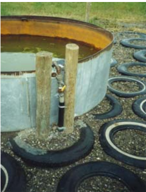
Ben Hansen's foundation of geo-grid and rubber tires filled with crushed gravel.
